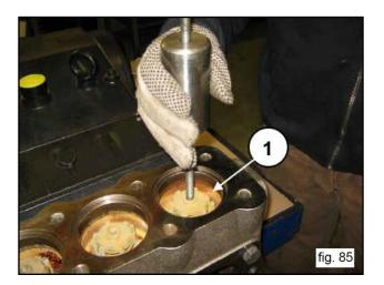
E) Extract the valves housing using tool #F27926900 (see mechanical drawings in par. 4.1) as indicated in fig. 86 and fig. 86/a.
